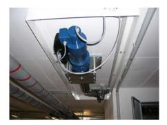
The actuator is mounted on the ceiling of the underground parking lot
