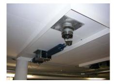
The thrust tube of the actuator is connected to the lever arm of the revolving glass door panel
